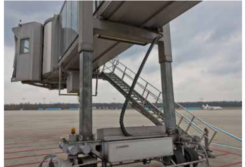
Passenger boarding bridges
